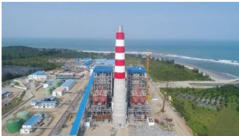
Figure 1. View of PLTU from above
